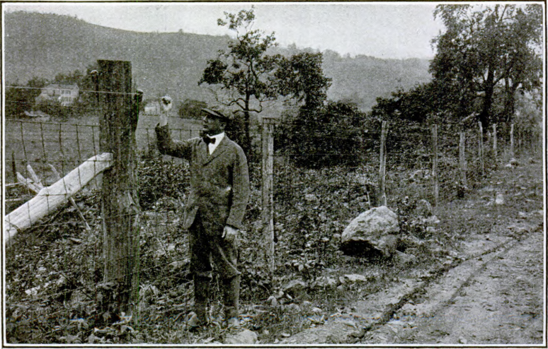
Fig. 5-34.—AERIAL LINE CONSTRUCTION, FENCE POST LINES.
